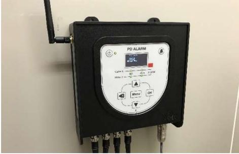
**PD Alarm** is an asset mounted device for indicating the presence of partial discharge in high voltage switchgear, ring main units (RMUs) and transformers. Designed for use in small substations, the instrument can activate local and remote alarms in addition to local indication.
