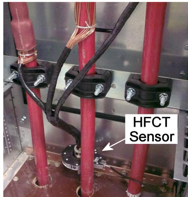
Figure 1: HFCT coupled to cable sheath
